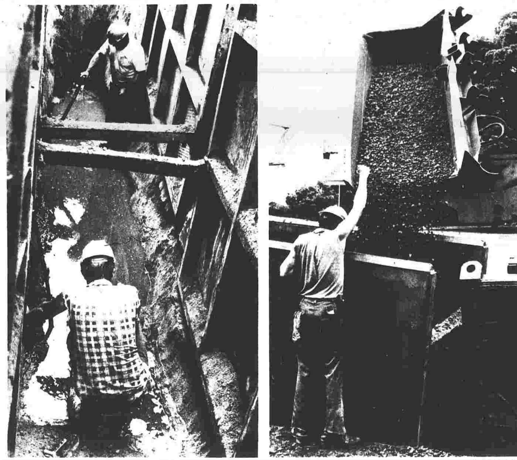
Work on Porter sewer
